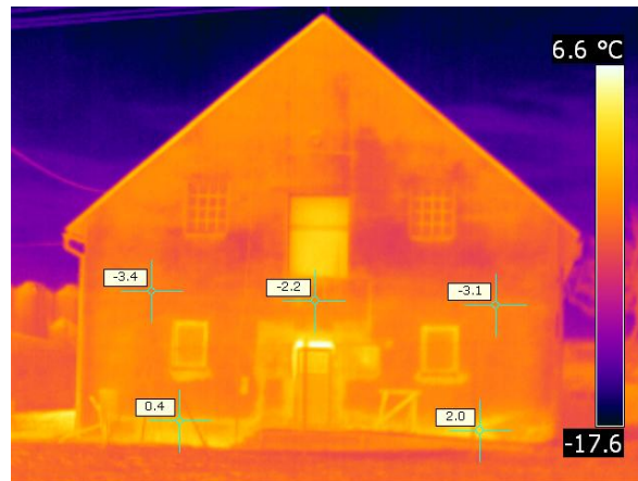
Fig. 7 South-east façade of piggery
